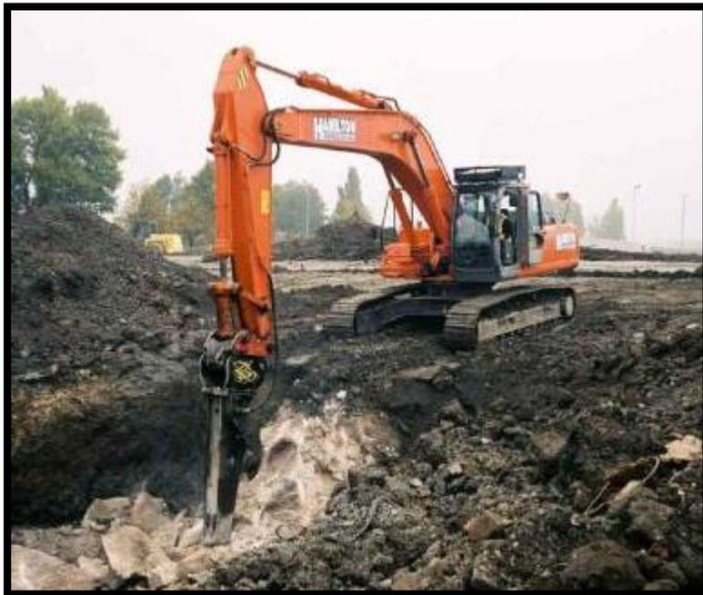
**Figure 6** – Hydraulic Breaker – Courtesy of Farley Plant Hire
